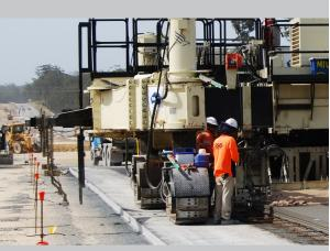
Electronic, no contact type, moisture proof, and proportional Sauer Danfoss (SD) steering and elevation sensors, as well as G&Z's own proprietary software version of the system provides precise steering and elevation accuracy and self-diagnostic capability.
